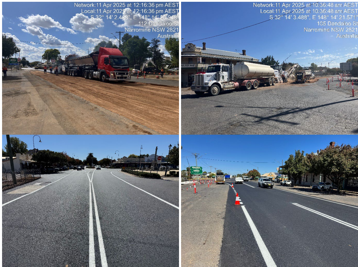
Figure 2: Asphalting works were completed at the Dandaloo Street Railway Crossing, Narromine
